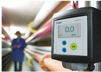
Installation & Commissioning Services.
